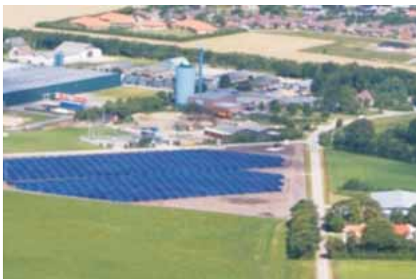
Figure 3. Aerial view of Gram District Solar Heating plant in Denmark (Foto: Arcon Solvarme)
