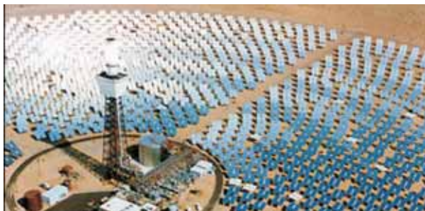
Figure 5. Aerial view of the Solar Two facility, showing the power tower (left) with storage tank next to it and surrounded by the sun-tracking mirrors [44]
