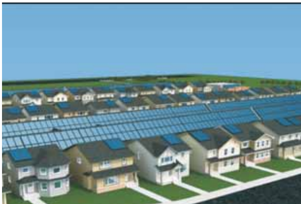
Figure 2. Okotoks district solar heating plant [37]
