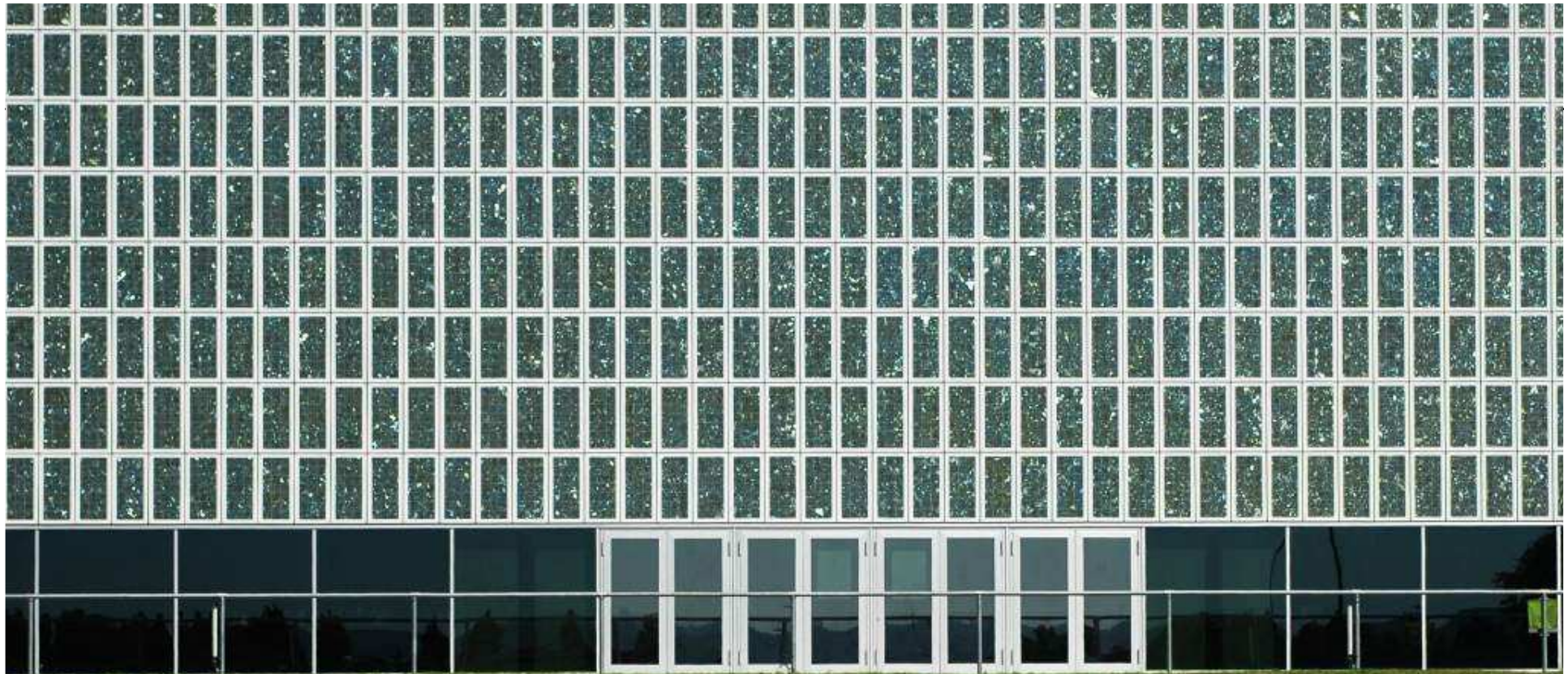
PV facade with green solar cells, sports stadium Tübingen
